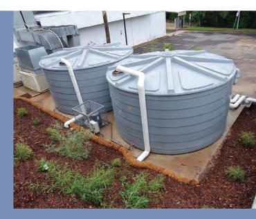
Two rainwater tanks at H Block. Kelvin Grove campus hold a total 68 000 litres (34 000 litres each tank).
