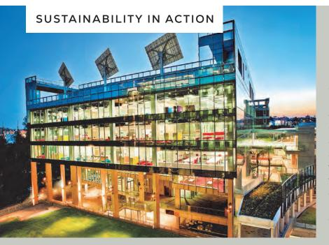
QUT's Science and Engineering Centre has a five-star Design Education VI certified rating from the Green Building Council of Australia. The building has a 200 kW solar PV array. Part of this array features three dual-axis trackers to align the modules throughout the day to achieve maximum power generation. When excess power is being generated, it can be fed into other buildings on campus.
